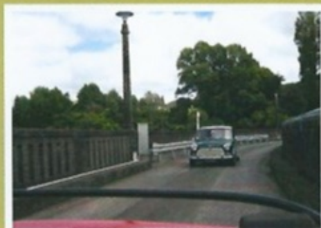
Day 1 Karapiro dam
